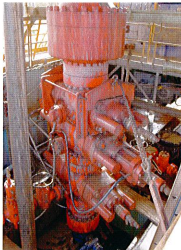
BOP (Blow Out Preventors) below the floor
