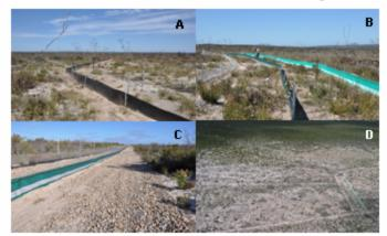
(A) Root impervious membranes and bunding were installed to prevent root-to-root trans mission and water associated spread of *P. cinnomomi*. The aim of the bunding was keep dean water out of the infested areas reducing risk of hydrological discharge of the pathogen and ensuring any contaminated water flows were channelled through geotextile filtrations ys tems.
