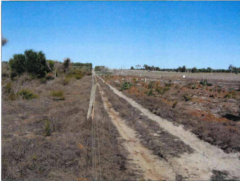
Plate C3: Williamson Road, Swan Coastal Plain. View shows artificial recharge system, injection bores in middle ground and water distribution pipe. Excavated ironstone is visible at surface. Williamson Road community is on left side of fence. Mining area behind the photographer, looking south. 25/5/06.
