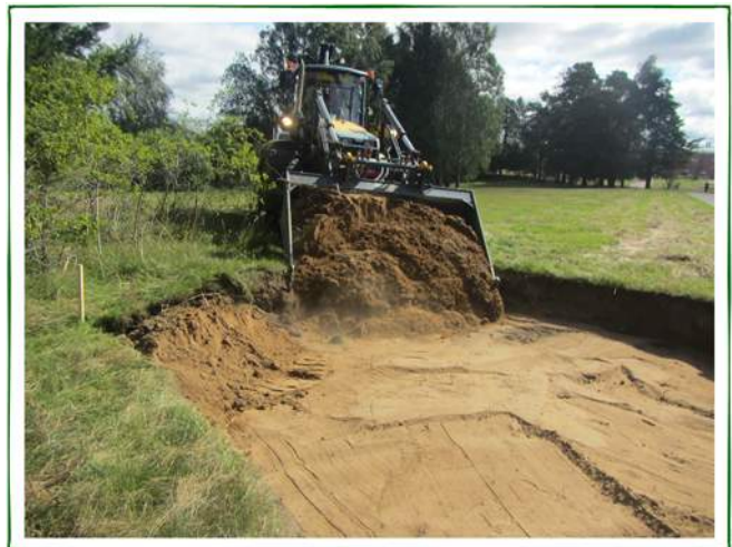
Moving sand with a backhoe © Niina Sallmén
