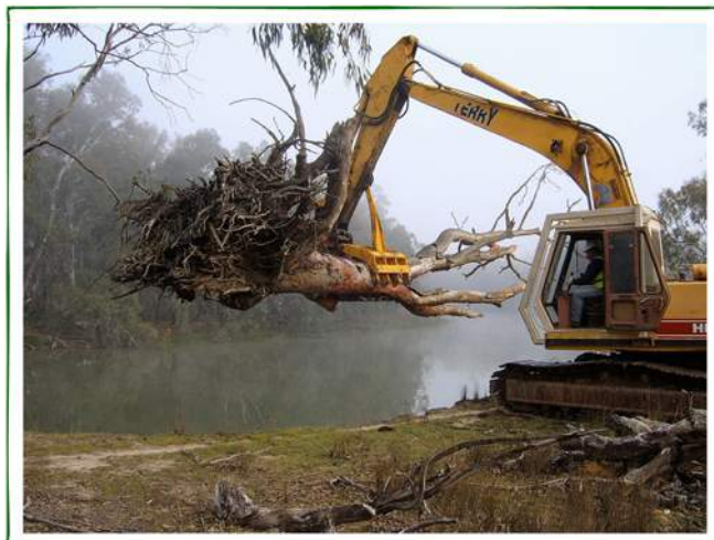
Installing woody habitat © Martin Casey
