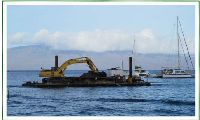
Dredging taking place at the receiving site
