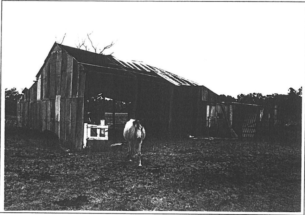
The barn, view looking north-west. Note the sheathing missing from the roof.
