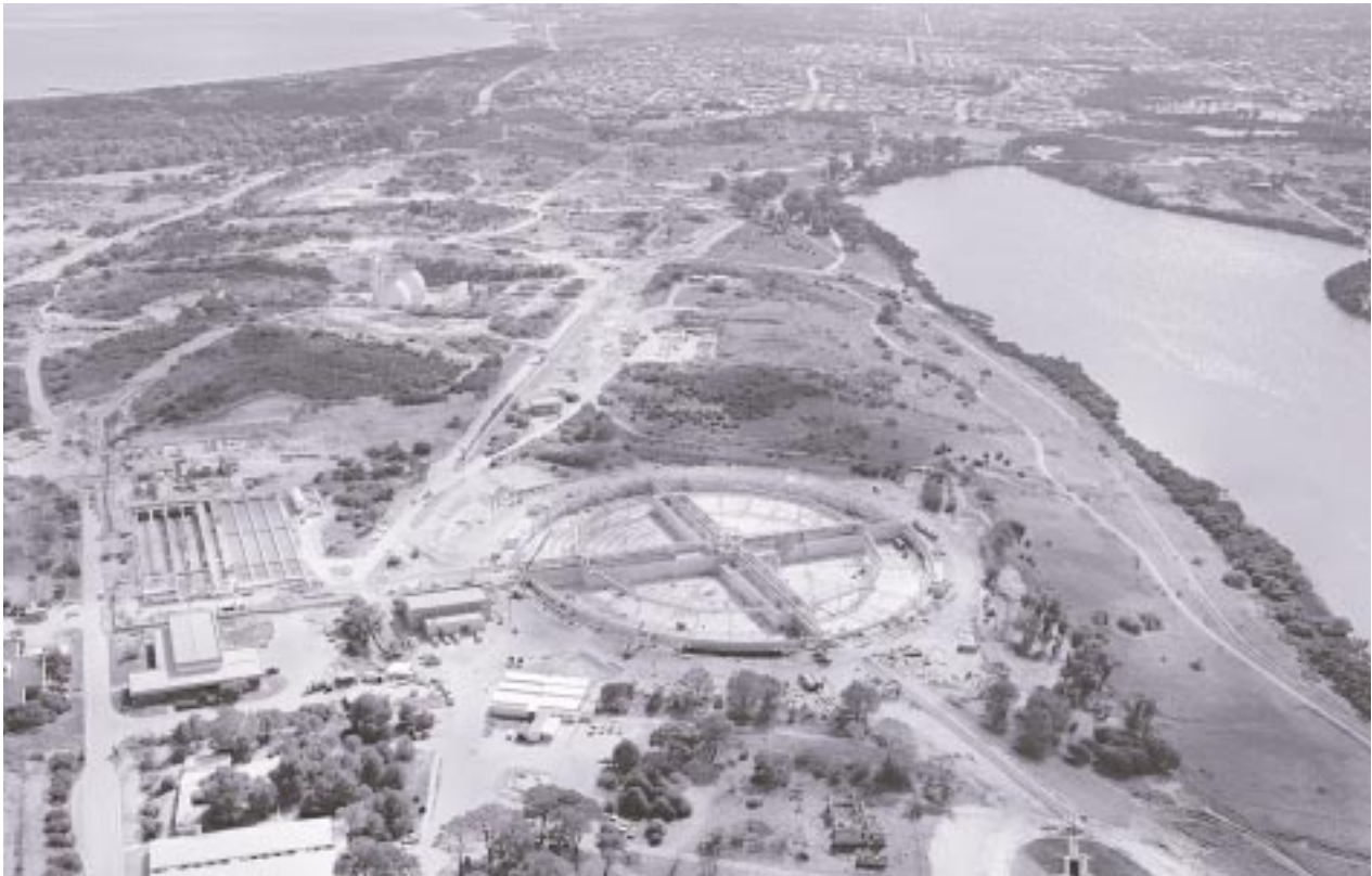
Perth's biggest wastewater treatment plant, at Woodman Point will be a key facility in the challenge to significantly increase the use of treated wastewater.
