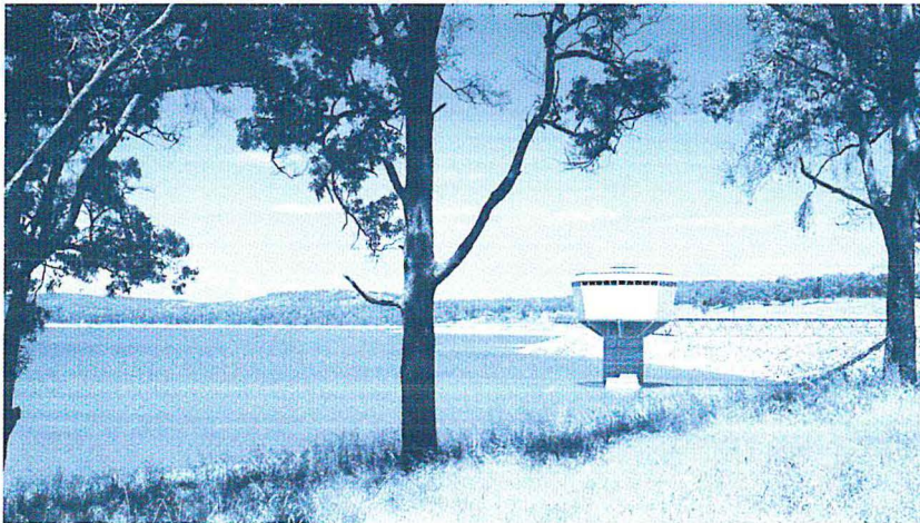
The new Harvey Dam supplies irrigation water to growers in a large area of the south west.
