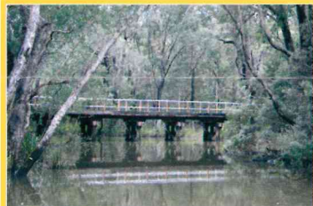
St John Brook Bridge You are now crossing St John Brook which joins the Blackwood River downstream. The old railway bridge is 80m long and was built by hand from local jarrah timber in 1909.
