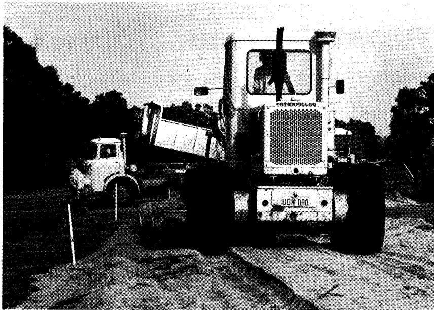
Sand mat fill over clay sub-base.
