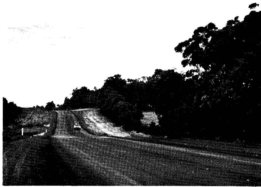
New construction prior to white lining.
