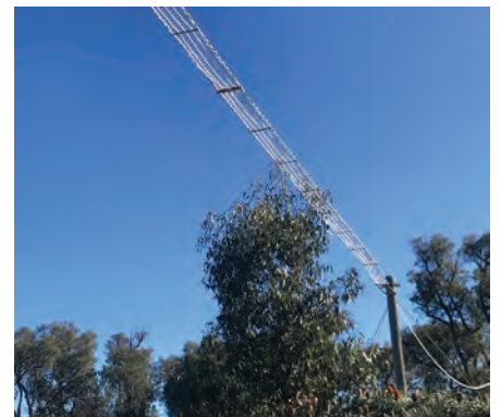
Top left The bridge was constructed at night to minimise disruption to traffic.
