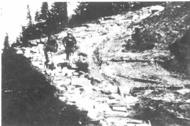
Attempts to control path erosion, Mount Rainier National Park.
