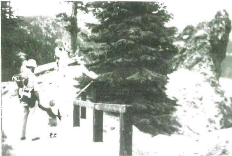
Poorly protected footpath, Crater Lake National Park. The ground 3m to the right of the child drops as a steep scree slope some 300m to the waters of Crater Lake (left).
