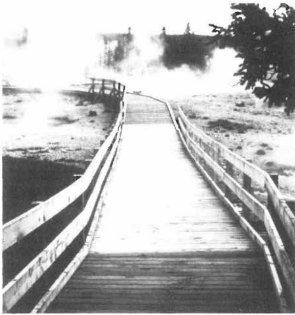
Boardwalks at Yellowstone National Park. Note experimental use of different timber treatments.
