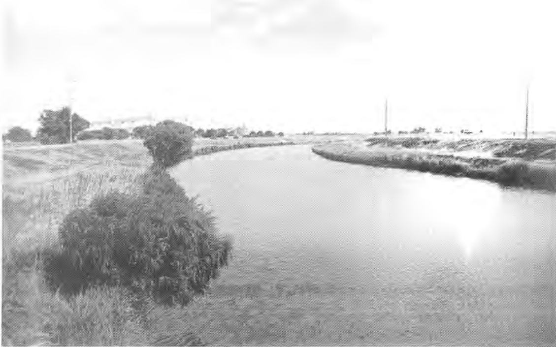
The relocation of the Preston River has resulted in artificial banks devoid of vegetation.
