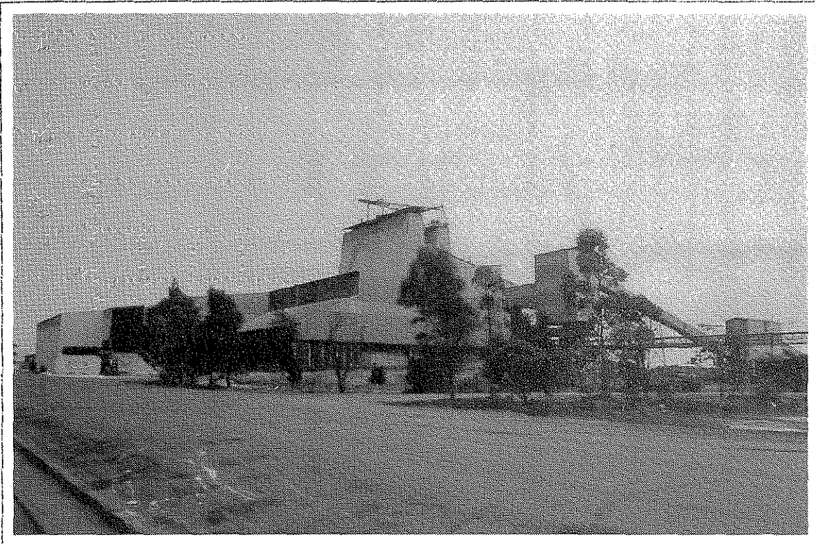
13. View of the Temco ferrosilicon smelter at Bell Bay. The enclosed conveyors on the right carry the raw materials. The furnace is in the centre, and product handling to the left. The baghouse is behind the furnace, obscured by the buildings.
