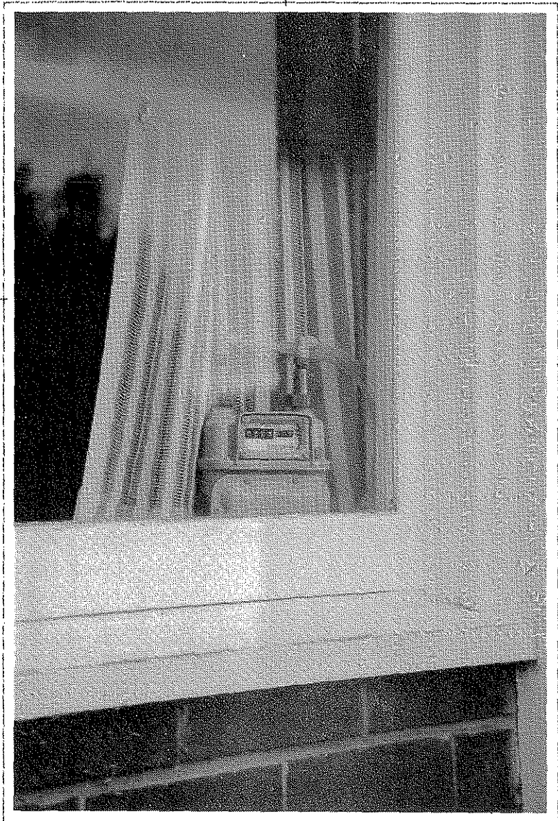
10. Close-up of the pump unit of the low volume sampler in the Headmaster's office, Snug Primary School.
