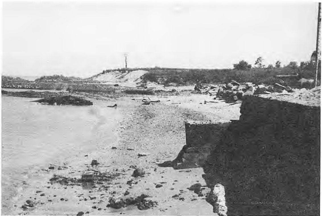
13. Townsite Foreshore with portion of reserve 31340 in the background. This area could be used as parkland or form an extension to the caravan park.
