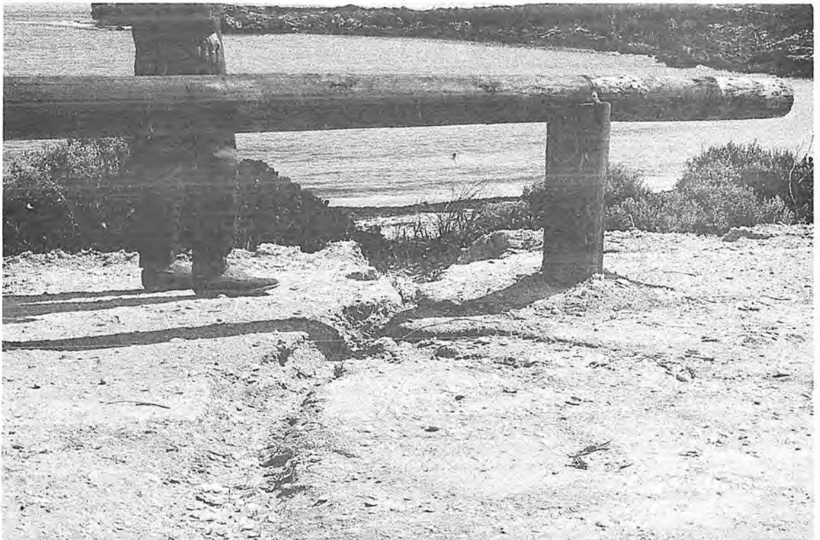
PLATE 6b : The carpark is already experiencing erosion in the form of gullying. There is also no formal access to the beach.
