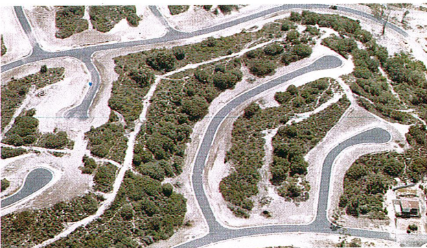
Subdivision on coastal sand dunes. A considerable area has been cleared for roads and other services.
