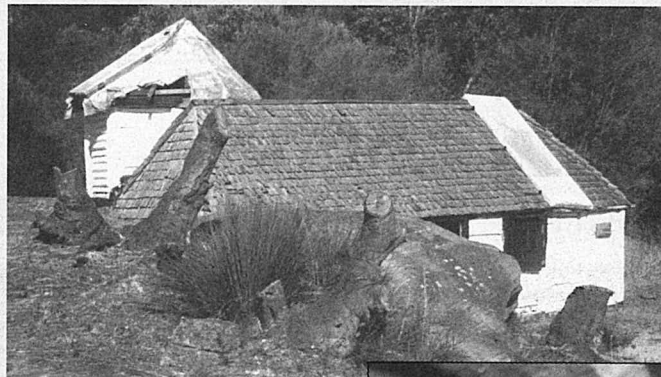
The Dawes Observatory was built onto the side of a rocky outcrop to help stabilise the instruments. The observatory dome was a wooden frame with canvas. It ran on a track with cannon balls. This reproduction can be found at Old Sydney Town (near Gosford, NSW)
