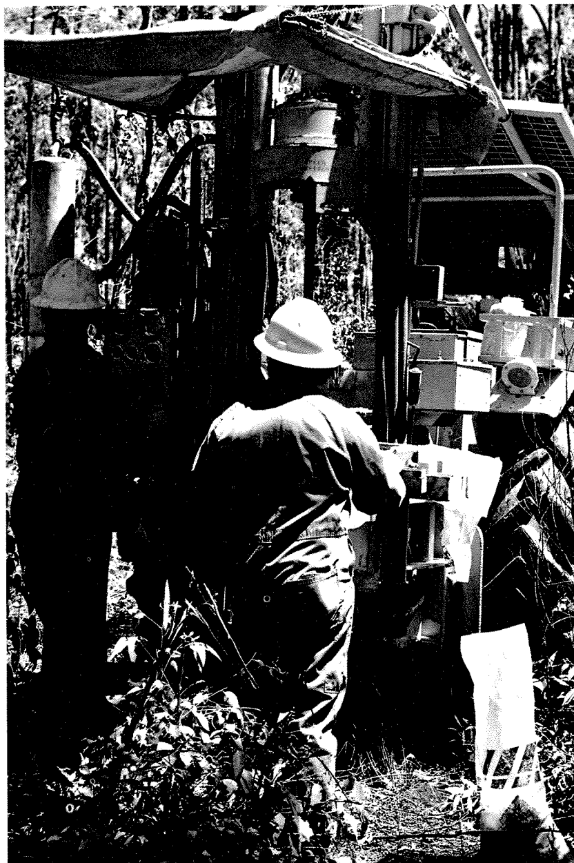
Figure 27. Tractor-mounted Edson vacuum drill in operation (Alcoa).
