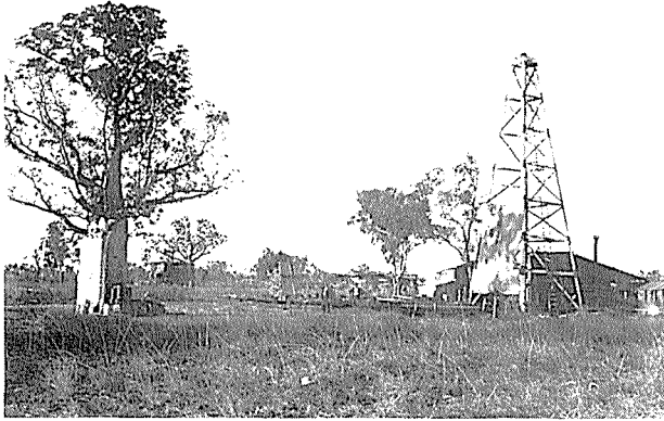
Figure 8. Drilling an artesian bore near Derby about 1910
