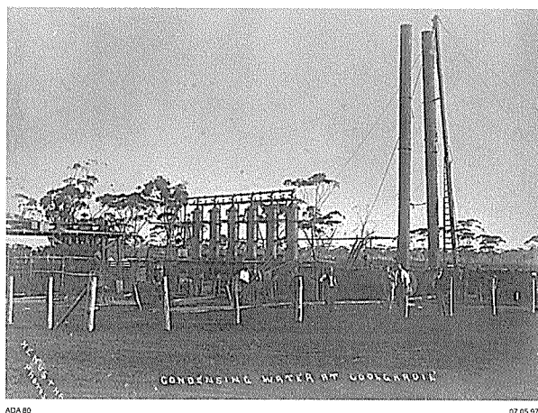
Figure 11. Condensers operating in Coolgardie about 1896
