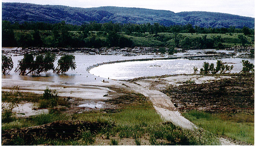
Ivanhoe Crossing in the 1960s, showing a sandbank deposited over the road and paperbarks growing upstream on a rocky shelf in the water.
