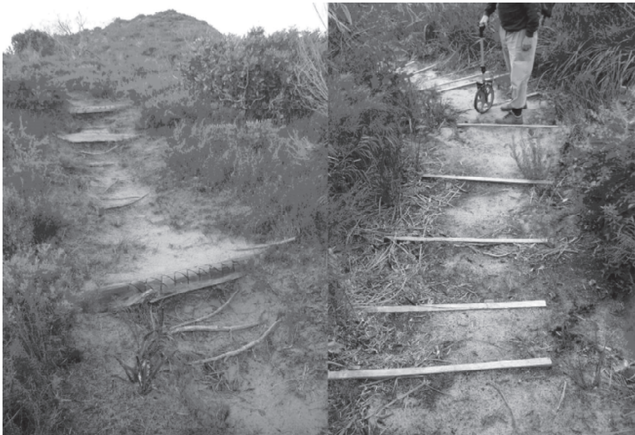
Figure 11. Water bars (left) with a tread space > 1m showing water erosion at the base of each bar due to the on trail waterfall created during surface water flow. Grouped steps (right) on a steep slope with a tread space of < 1m, show no signs of water erosion or soil movement. Bibbulmun Track in WCHNP
