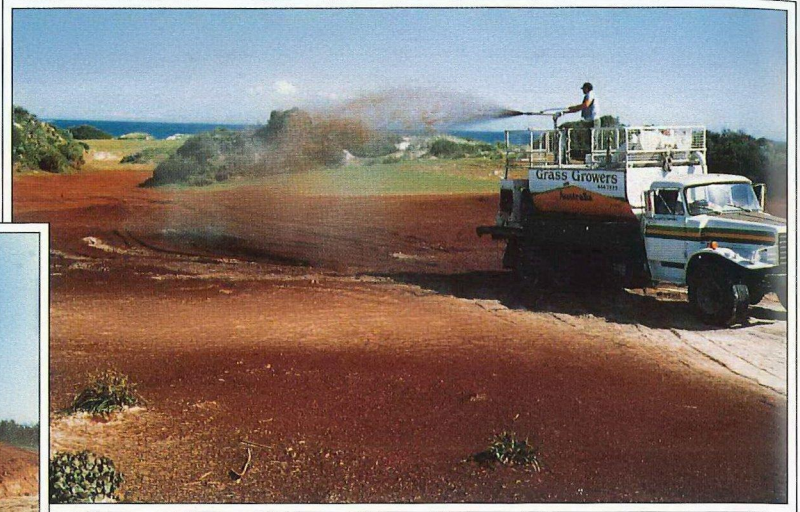
Figure 47. Applying hydromulch on development sites by machine (photo: Grass Growers and Australian Sandstill)
