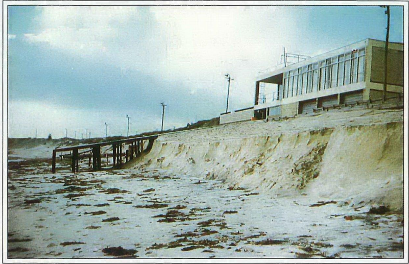
Figure 28. Cyclone Alby caused severe wave erosion which threatened the North Cottesloe Surf Lifesaving Club (photo: J. Broun)
