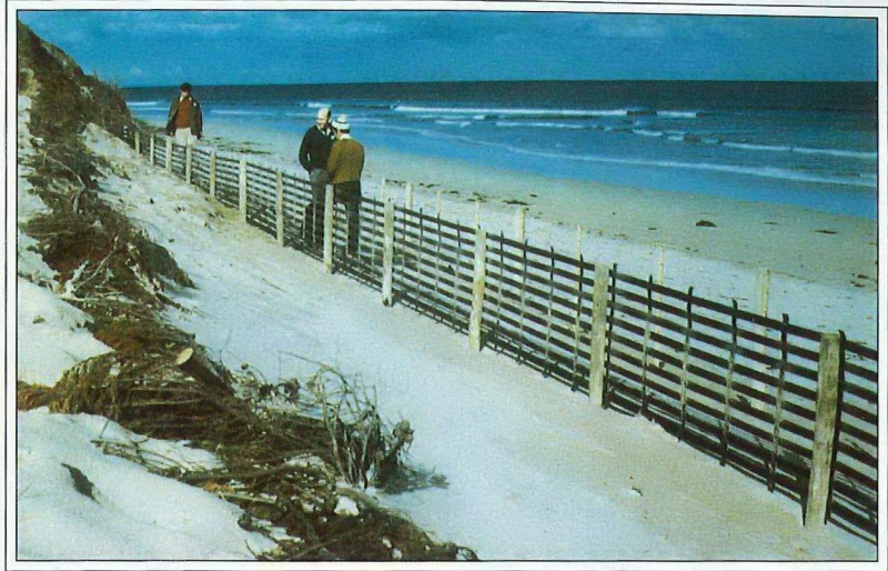
Figure 39. A Paraweb® sand trapping fence (photo: J. Broun)
