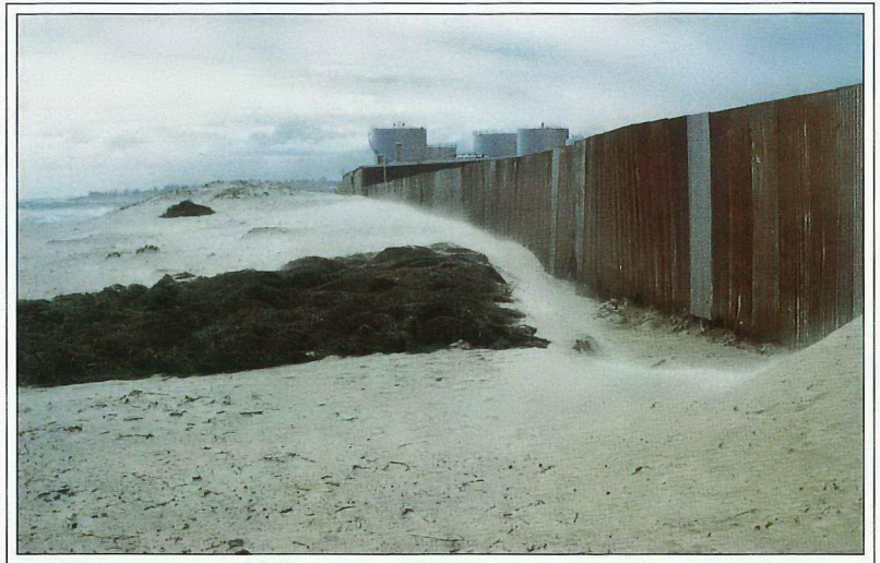
Figure 35. Wind erosion can occur due to wind eddying around buildings and structures. This problem area is being temporarily stabilised with brush (photo: J. Brown)
