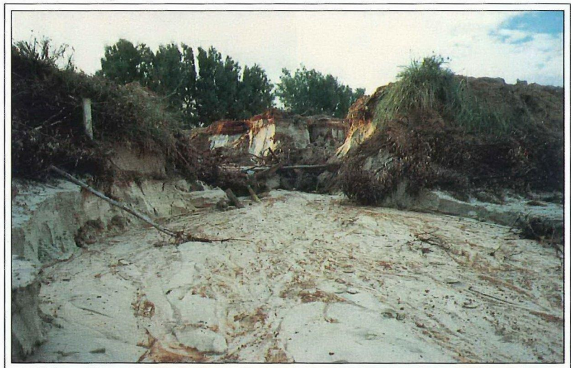
Figure 30. Erosion of the foredune at Geraldton was caused by runoff from the adjacent caravan park (photo: J. Broun)
