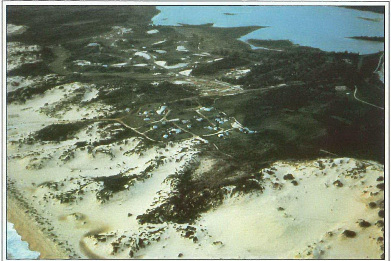
Figure 24. Blowouts threatening the coastal settlement at Preston Beach (photo: S. Chape)
