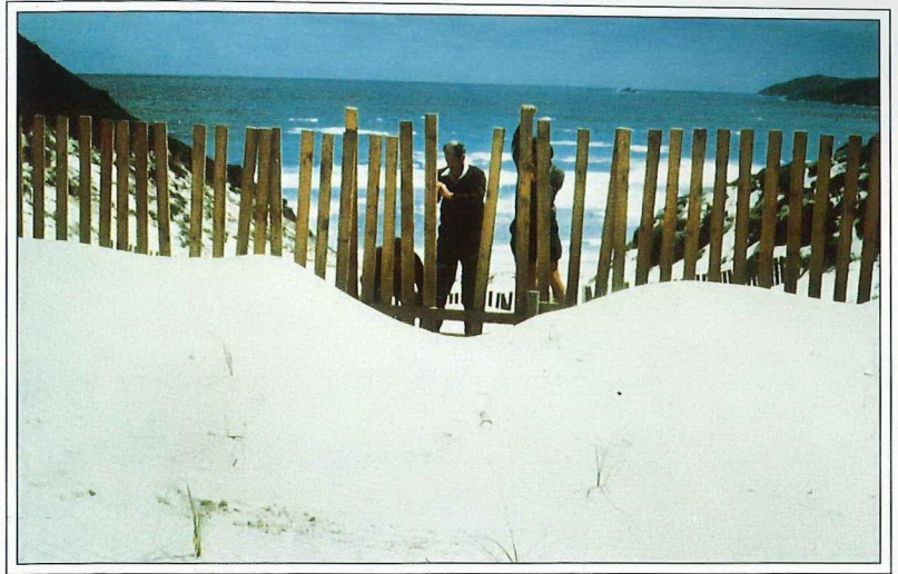
Figure 42. A sand trapping fence created across a blowout by driving wooden slats into the sand (photo: J. Grasby)
