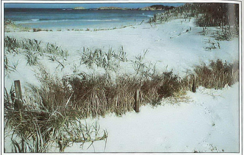
Figure 40. A sand trapping fence constructed with brush woven through wire (photo: J. Broun)
