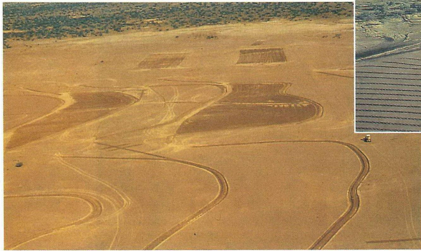
Water ponding and cultivation trial site in the Carnarvon area. The tractor indicates the size of these motorgrader-built ponding banks.
