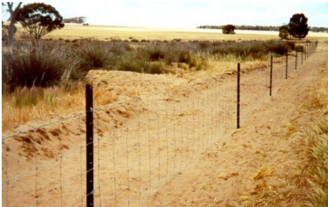
Fencing provides a means of excluding stock from waterways, decreasing erosion associated with grazing and trampling, and allowing native species to regenerate
