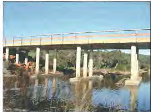
Photograph 4: The new Port Gregory Road bridge minimised disturbance to flow.
