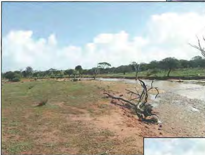
D grade foreshore: Deposits of sediment are accumulating along the river and the river channel is widening and eroding back into farmland.
