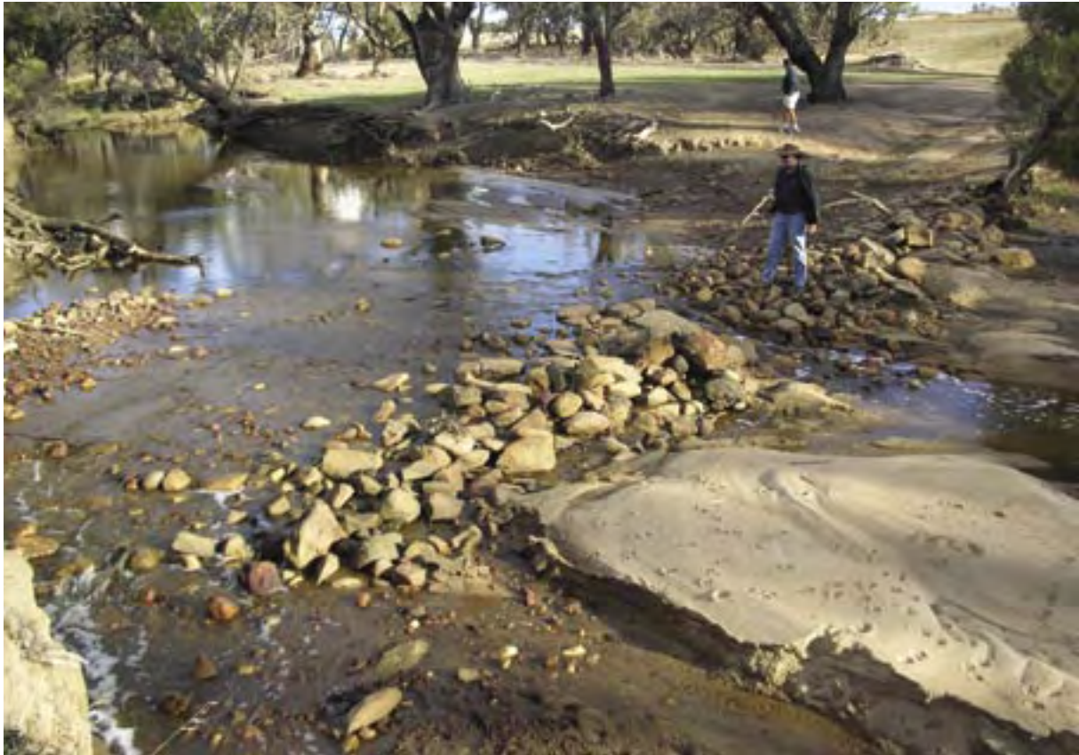
Photo 11 Vehicle crossing which doubles as a riffle
