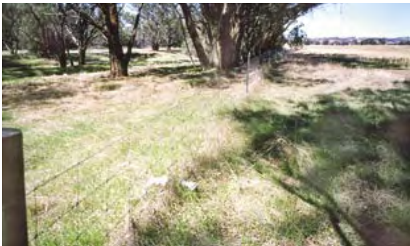
Fence in good condition
