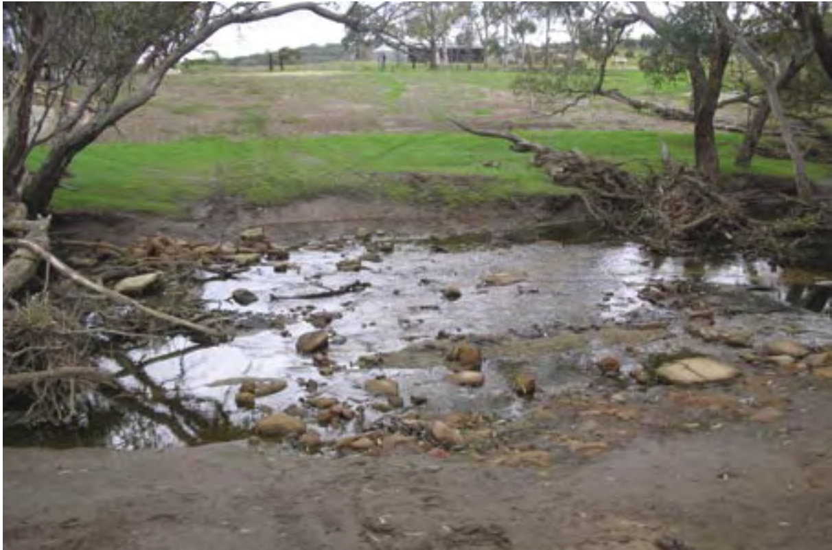
Photo 6 Farm crossing stabilised with field stone
