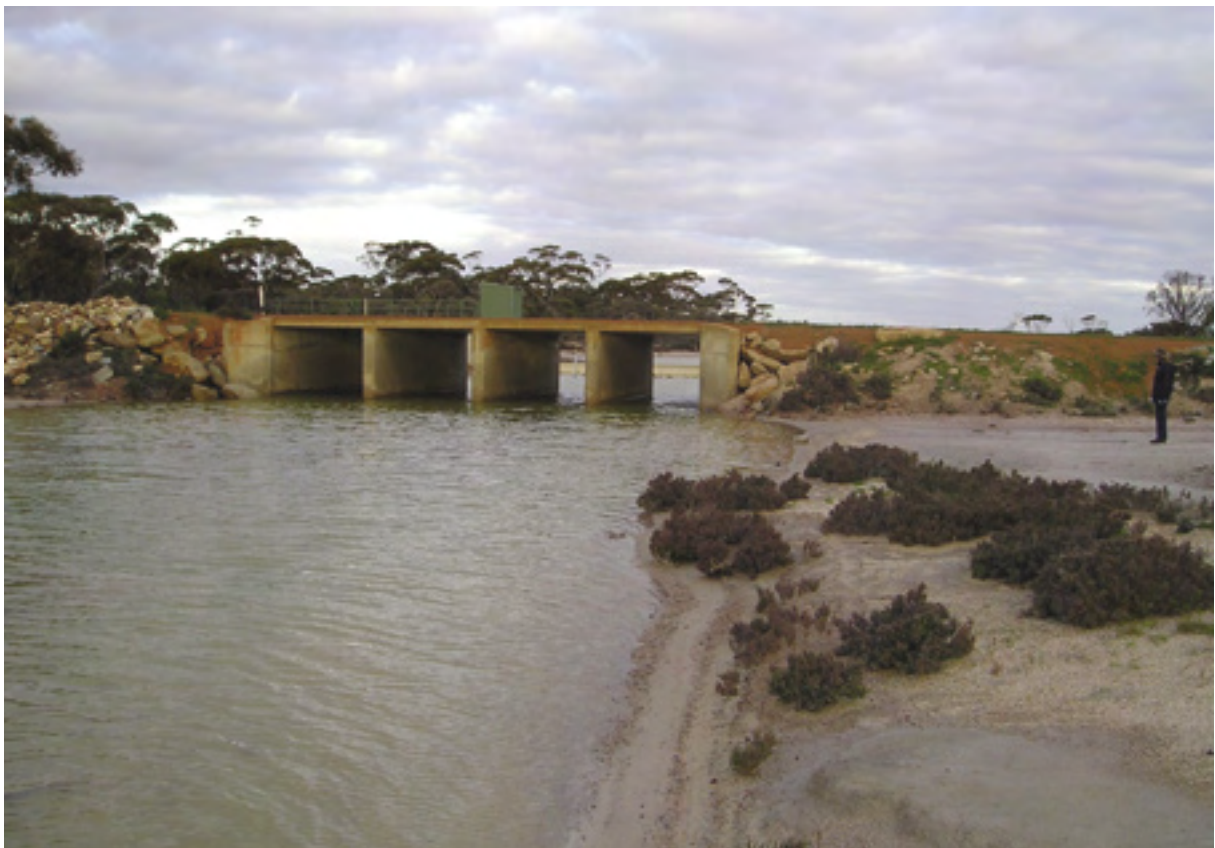
Photo 8 Box culvert structures for Kwolyin East Road
