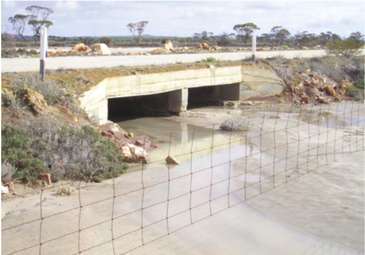
Photo 13 Box culvert on the Shackleton Road
