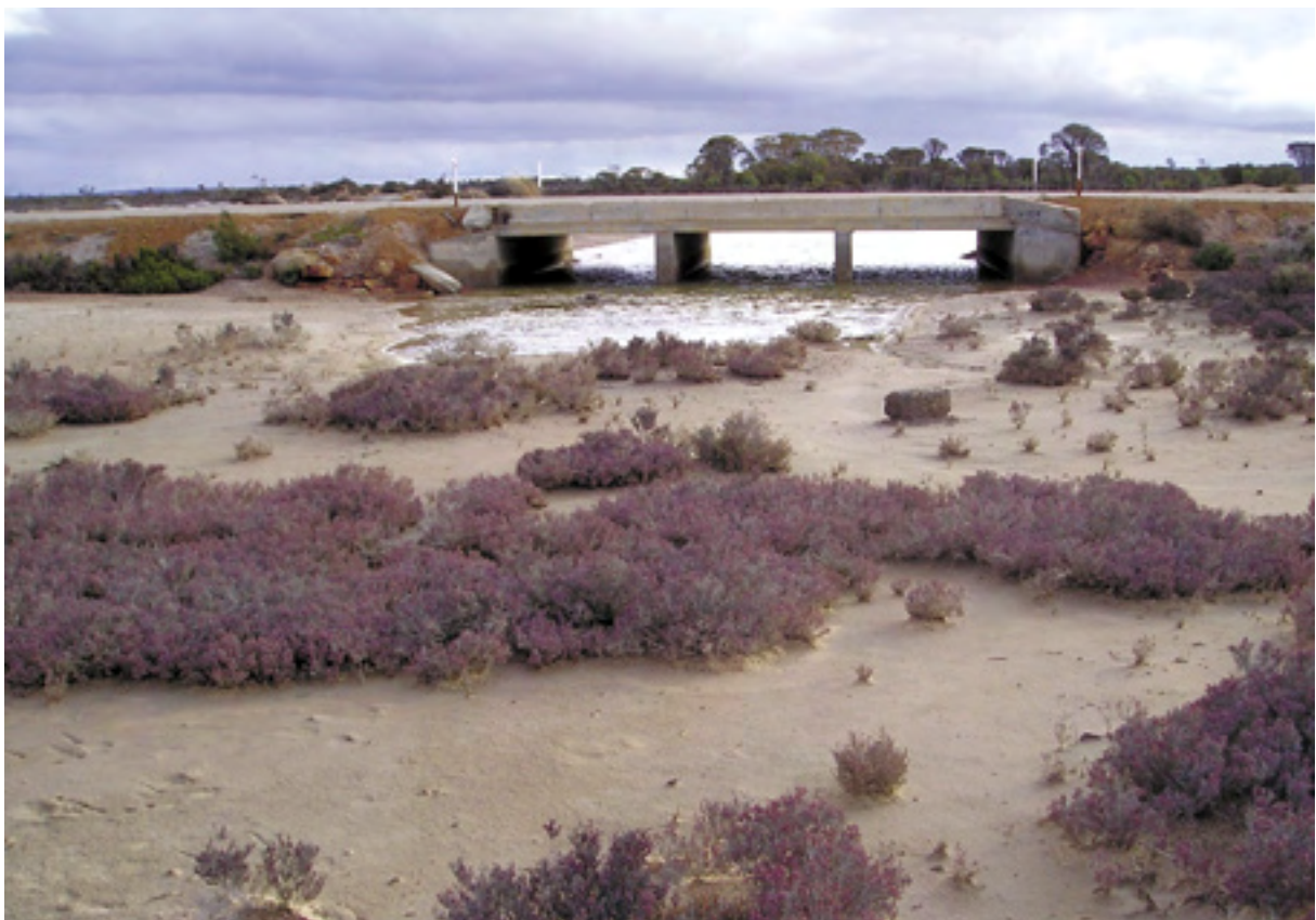
Photo 27 Box culverts on the Ardath-Yarding Road
