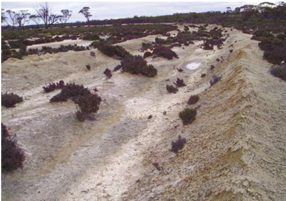
Photo 31 'W-drain' constructed for surface water management
