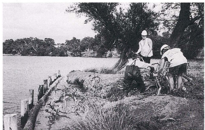
Erosion control works at Ron Courtney Island, 1995.
