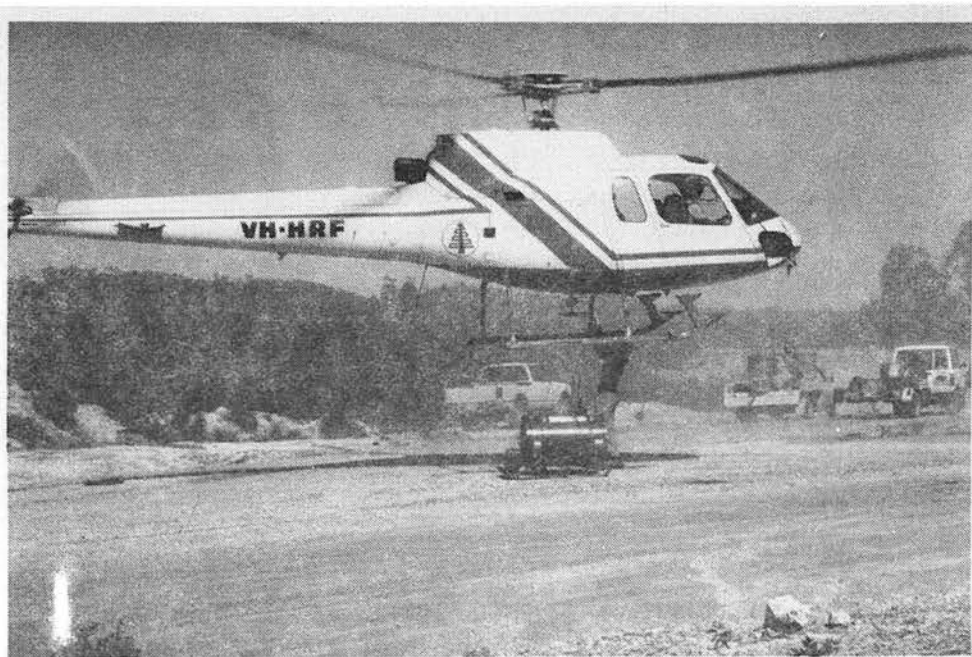
FIGURE 6. LIFTING STRAP BEING HOOKED TO HELICOPTER.
