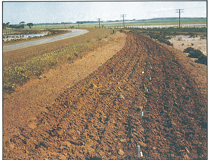
Saltbush planted on the road verge near Dumbleyung will highlight the verge at night and act as a cushion for motoring accidents.
