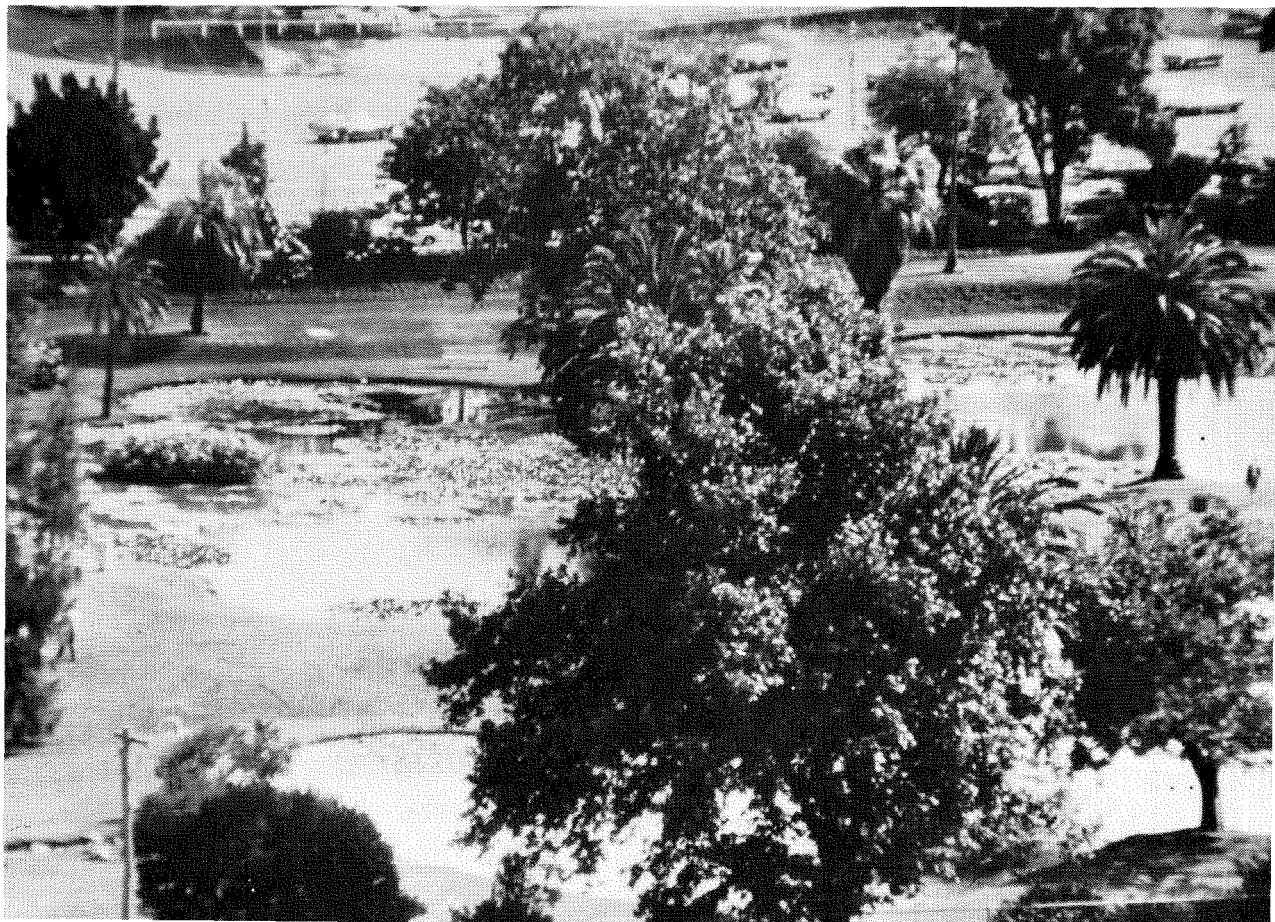
Queen's Gardens, Hay Street east—site of Perth's first clay pits
