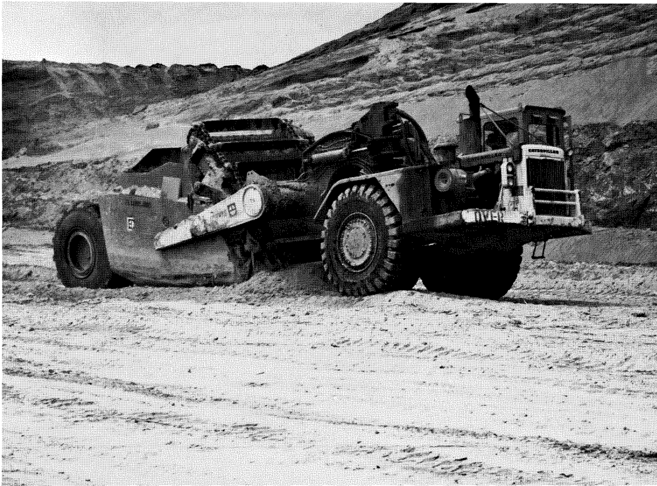
Mining sand at Allied Minerals' Eneabba pit.
