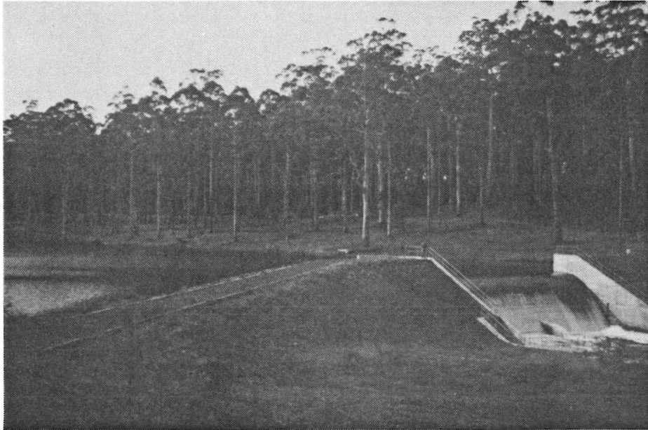
A view of Big Brook Dam looking in a north-easterly direction. The photograph was taken in June 1988 soon after the spillway overtopped. The main day use area can be seen in the background.
