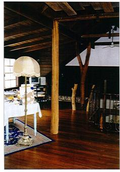
Wandoo in use – floorboards, roof timbers and support poles. The floorboards are recycled, the rest was cut from the property. "Northumbria", Boyup Brook. Photo, Julian Sumner.
