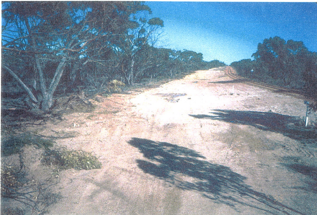
Plate 6. Track along railway line showing extensive clearing and widening to relay sleepers and replace culverts. Note total clearance of vegetation between railway line and access track and material push up into reserve.
