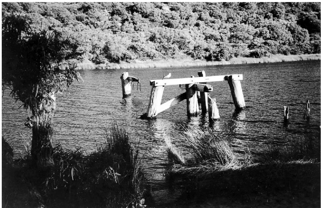
Many inlets have, in the past, facilitated transport of agricultural produce. - Torbay Inlet - (CoA).
