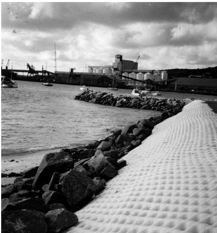
Hindsight indicates that provision of an adequate setback at the time Esperance was established, may have avoided the need for shoreline revetment and costly beach renourishment.
