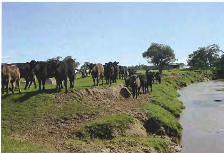
D2 Grade foreshore, showing a major cause of problems in the catchment – unrestricted stock access.
