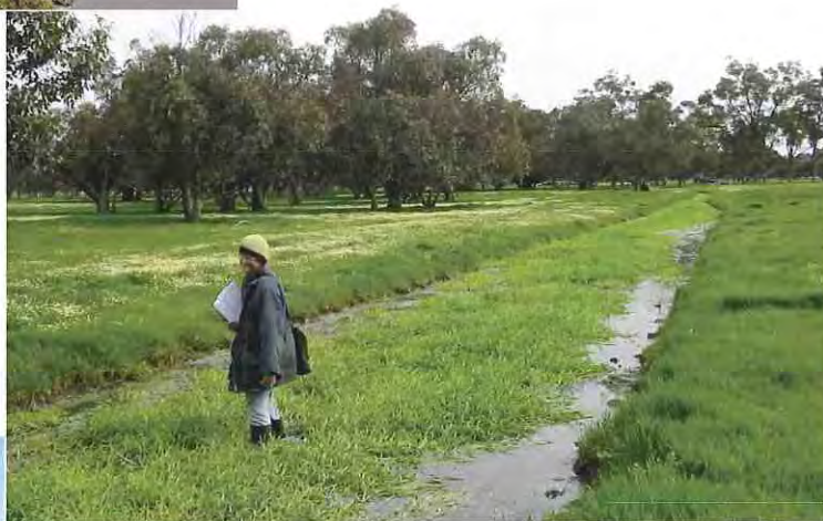
D3 grade foreshore. This drain has no remaining fringing vegetation, and is heavily infested with exotic species. The banks are stable however, and erosion is not a significant issue in this part. It is important to ensure invasive weeds are well managed to minimise potential problems downstream.
