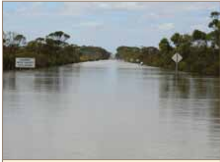
Flooding along the Newdegate to Pingrup Road that occurred in January 2006. Photo – Natalie Nicholson/DEC Katanning
