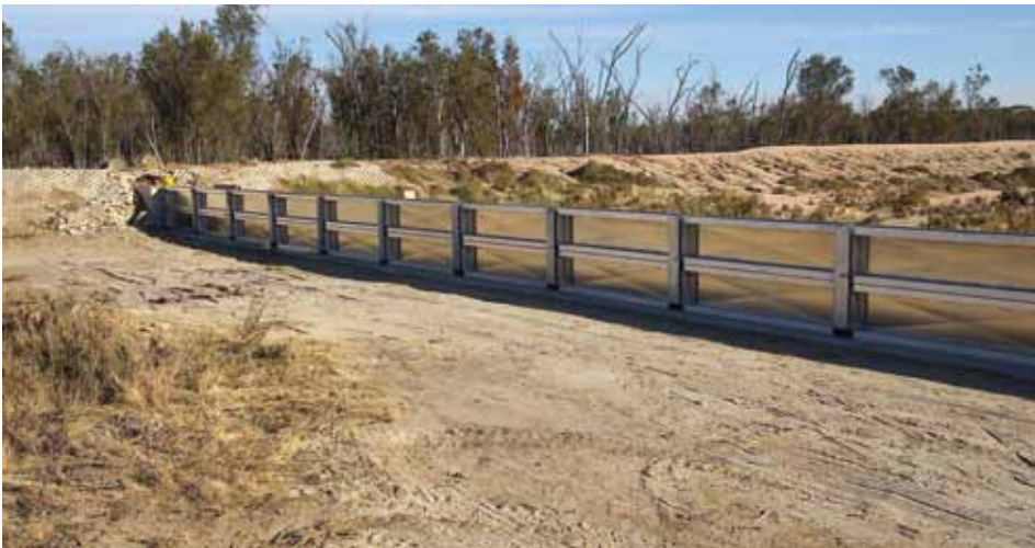
Figure 11. Controlling surface water flows into Toolibin Lake using a separator gate. It captures and diverts low volume, high salinity flows, preventing them from entering the wetland. Photo – L Mudgway/DEC.
