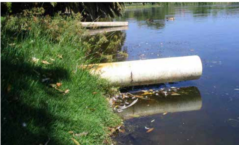
Figure 1. Pipes discharge stormwater into Lake Monger, Perth. Photo – L Mazzella/Department of Water.
