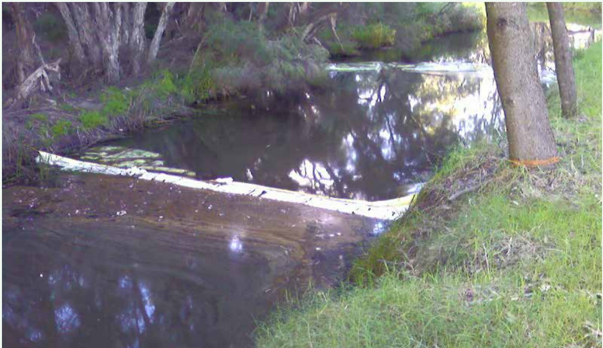
Figure 43. The hydrocarbon interception system installed by the City of Stirling to protect Herdsman Lake from hydrocarbon contamination carried in with stormwater from the surrounding light industrial area. Photo – Oleology.
