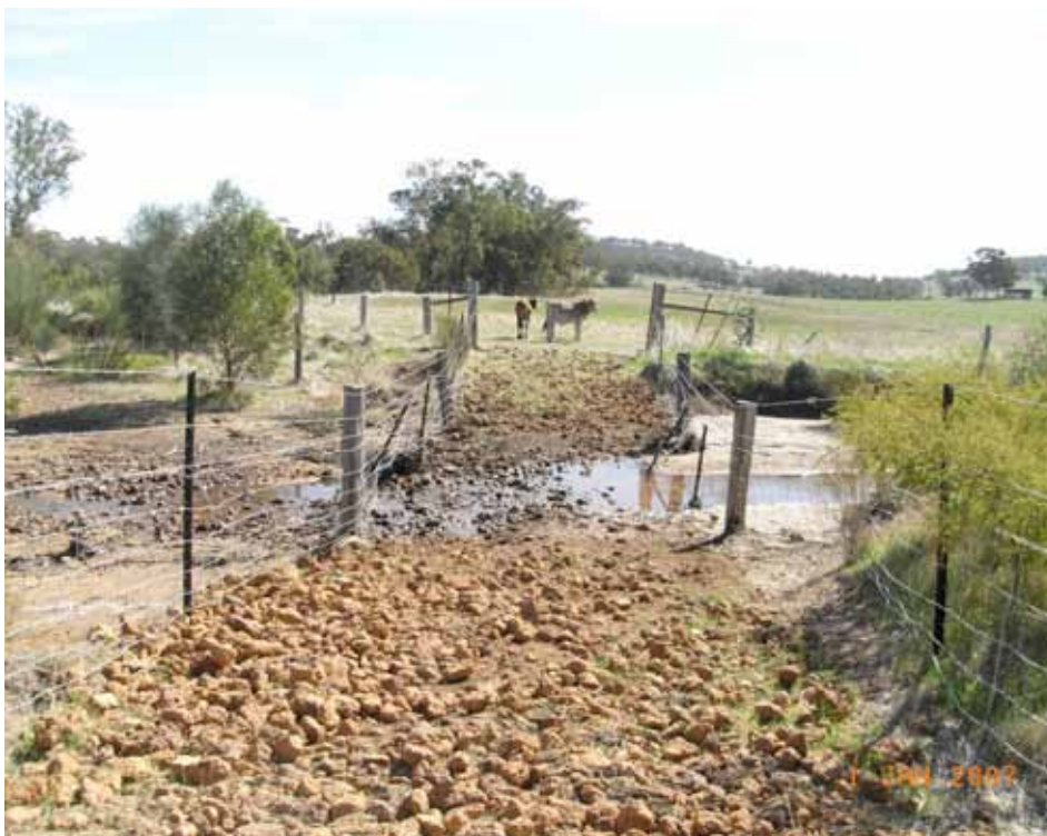
Figure 32. A fenced laneway with a compacted rocky ramp allows cattle to access and cross a waterway, but minimises damage at the site and protects the rest of the waterway. Photo – R Thorpe/Chittering Landcare Centre.
