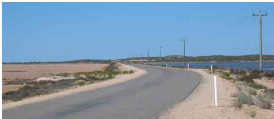
Figure 13. The causeway across Lake McLeod in the Gascoyne region prevents the spread of surface water across the bed of the wetland. Photo - A Lam.
