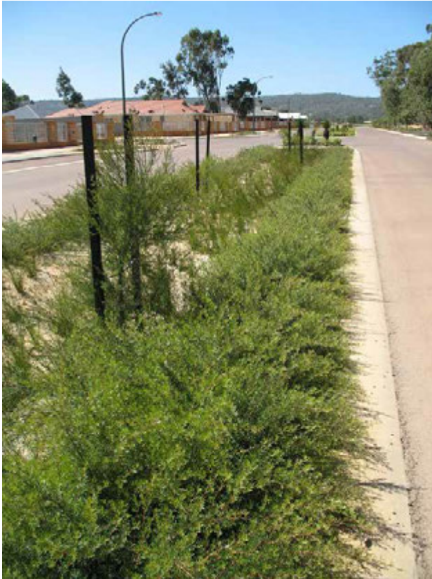
Figure 36. Vegetated swales and flush kerbs capture and infiltrate rainfall along the length of this road in The Glades, Byford. Photo – courtesy www.newWAterways.org.au .
