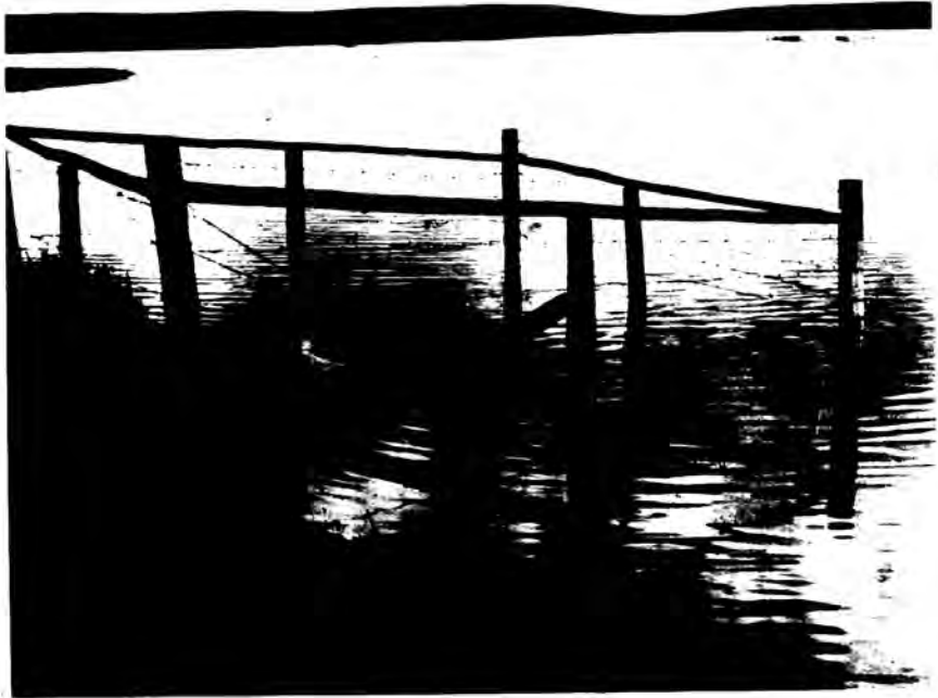
Fig. 4. Overflow structure on D-area Lake.
