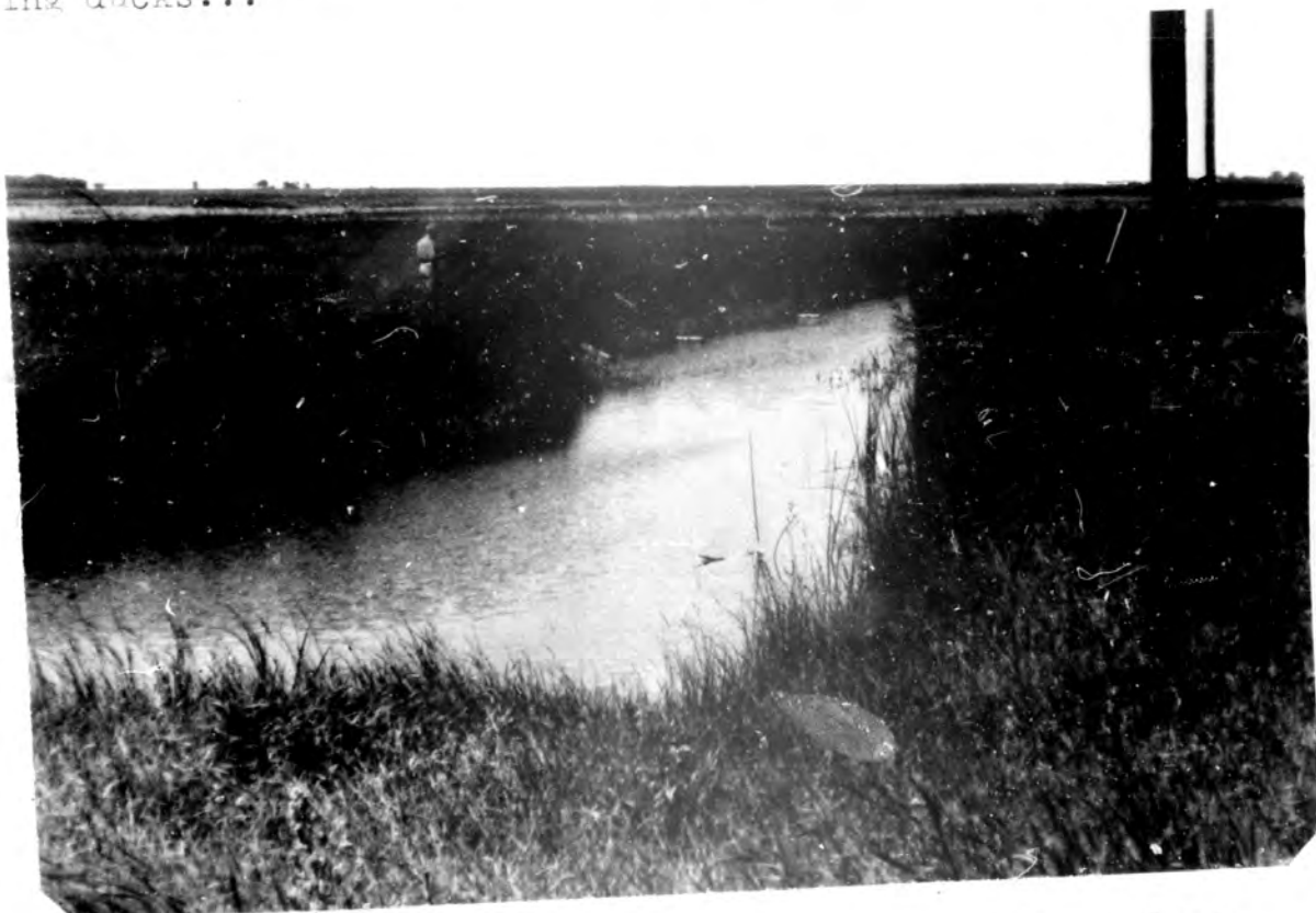
Figure 21 ...than were ditches with grown over edges.
