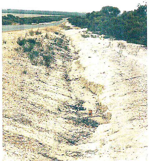
Control runoff from cleared areas to avoid erosion. (Photo by K Vaux)
