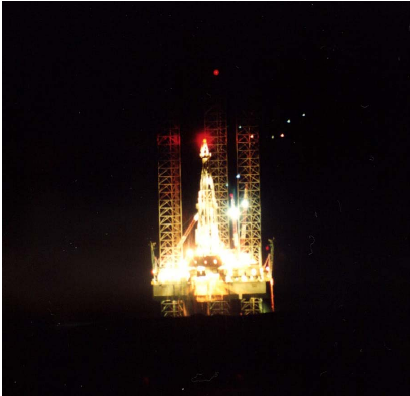
Plate 5.3: The drilling rig Enasco 56 light field photographed from 1.5 km, 70-200 mm zoom lens
