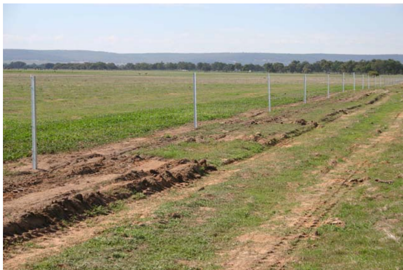
Figure 2: The new northern boundary fence installed at Bootine Nature Reserve.
