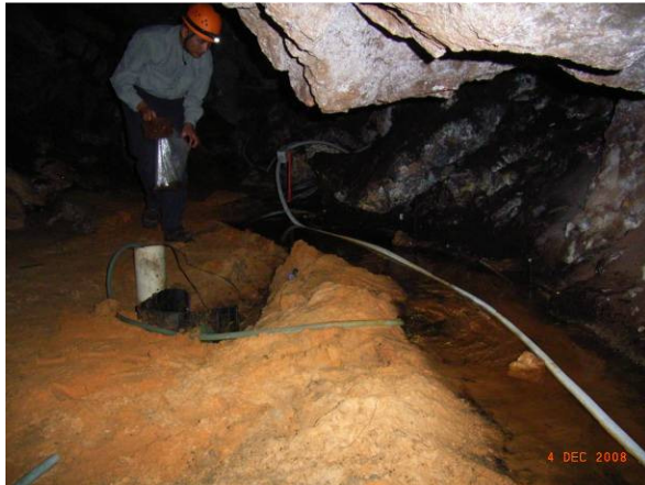
Plate 1. Main pondage in Cabaret Cave with pipe work and showing water in the liner (December 2008).
