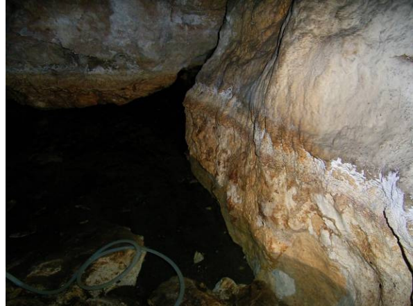
Plate 4. Main pool in Water Cave, showing water level below historical water marks on the exposed rock face (Oct 2007).
