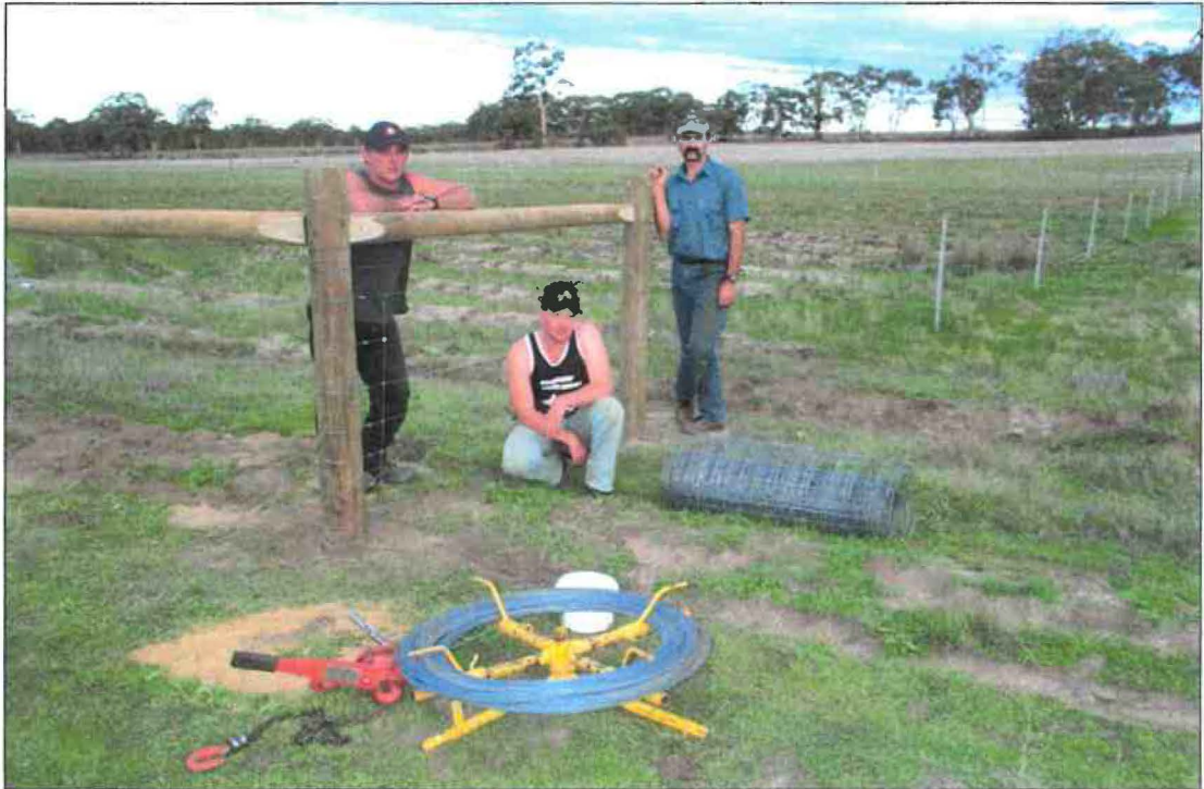
DCLM staff completing fencing work on “Emu Farm” paddock revegetation site.
