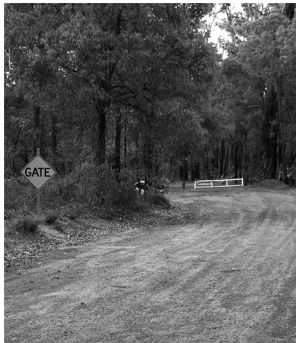
Diagram E2.8 Emergency access ways may be used to link up with roads to allow alternative ingress and egress during fire emergencies. Emergency access way gates must not be locked. (Ref. P2, A2.8 and A2.10)
