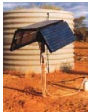
Solar powered water pump.
