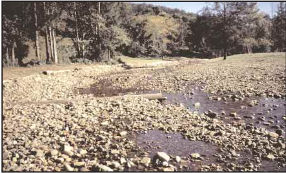
Figure 23. Bendway weirs used to move the thalweg from the bank to the centre of the channel on Pappinbarra Creek, a tributary of the Hastings River, in New South Wales.
