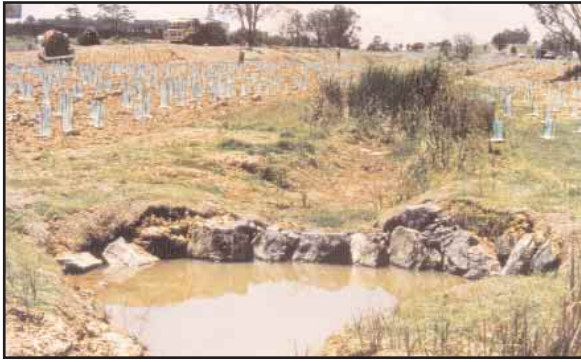
Figure 2. Rock-boulder structures on Eastern Creek (Sydney) (by Wal Hader).
