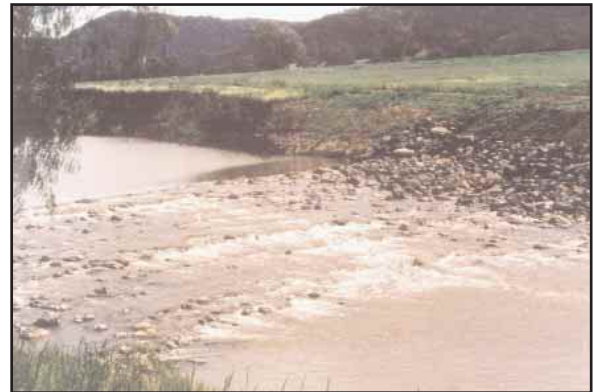
Figure 1. Rock grade-control structures in Bell River (Wellington, New South Wales) have been constructed to protect the bed, but also incorporate a low gradient to allow fish passage (figure by Wal Hader).
