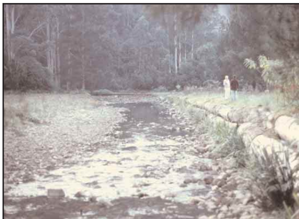
Figure 34. Logs used as bank protection on Pappinbarra Creek, a tributary of the Hastings River, northern New South Wales. Logs are about 0.4 m diameter.
