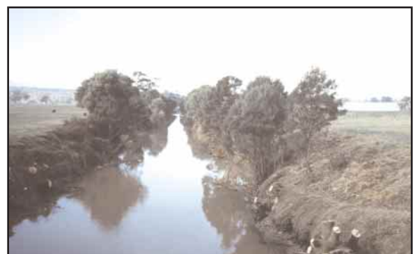
Figure 39. Twenty kilometres of the Moe River in Victoria has been straightened and original meander bends have been backfilled, making reinstatement of meander cut-offs uneconomical.
