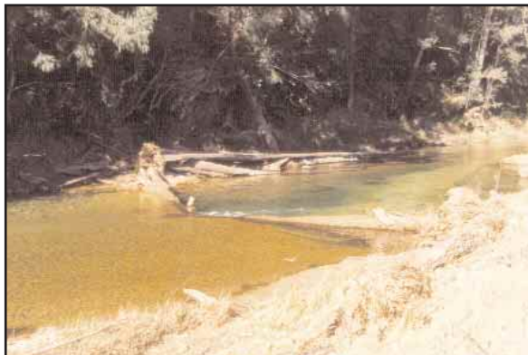
Figure 12. A Schauberger sill (flow from left to right). Note that the apex of the sill is the lowest point, and is pointing upstream. As a result, the flow is concentrated in the centre of the channel, and there is a deep scour pool downstream of the structure (photo by Wal Hader).
