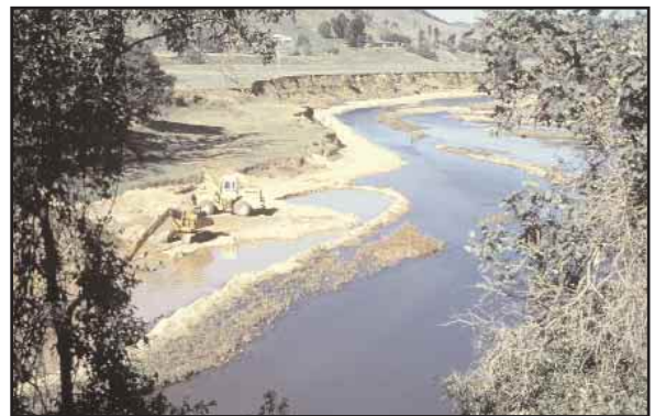
Figure 55. A sand extraction operation on the Mary River in Queensland.
