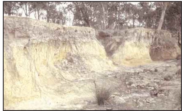
Figure 60. The roots of the trees growing on the banks of this gully do not penetrate deeply enough to stabilise the toe of the bank.
