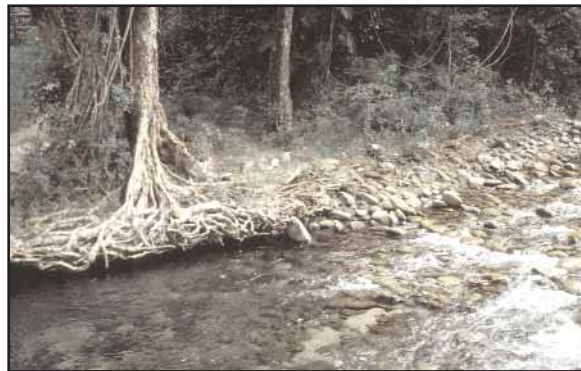
Figure 63. Undercutting of the bank in Babinda Creek in far north Queensland.
