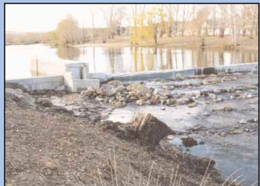
Figure 48. Macdonald's Weir rock-ramp showing dislodged downstream rocks (photo by John Harris).
