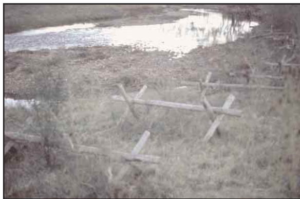
Figure 18. Jacks at the Gloucester River site, 5 years after installation.
