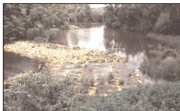
Figure 46. A zigzag fishway, with transverse ridges of rock that effectively reduce the slope of the fishway (photo by John Harris).
