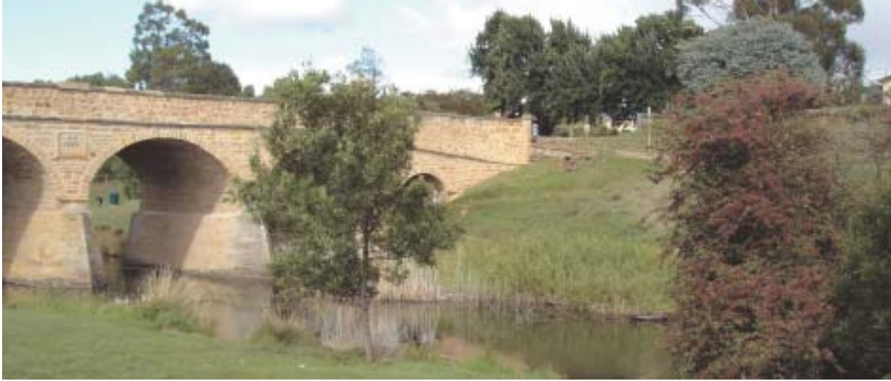
Willow removal has taken place along the Coal River to protect the historic Richmond Bridge.
